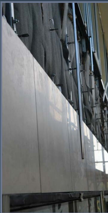
Selina Gold limestone facade mounted with galvanized iron fixing elements
